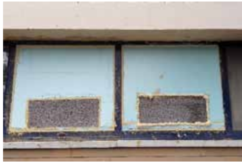
Figure 16. Thermal insulation test of CMU (exterior view). March 2014.
