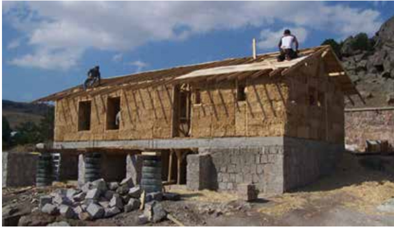
Figure 3. Straw bales used as infill wall at the Kerkenes Eco-Center [19].
