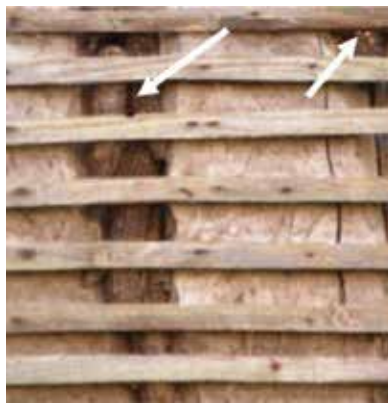
Figure 1. A traditional external tabique wall showing corncob as a filling material.
