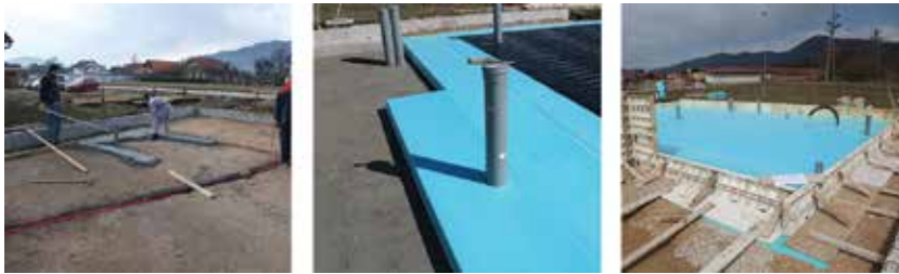
Figure 1. Example of extruded polystyrene (XPS) insulation boards used under a foundation slab [6].
