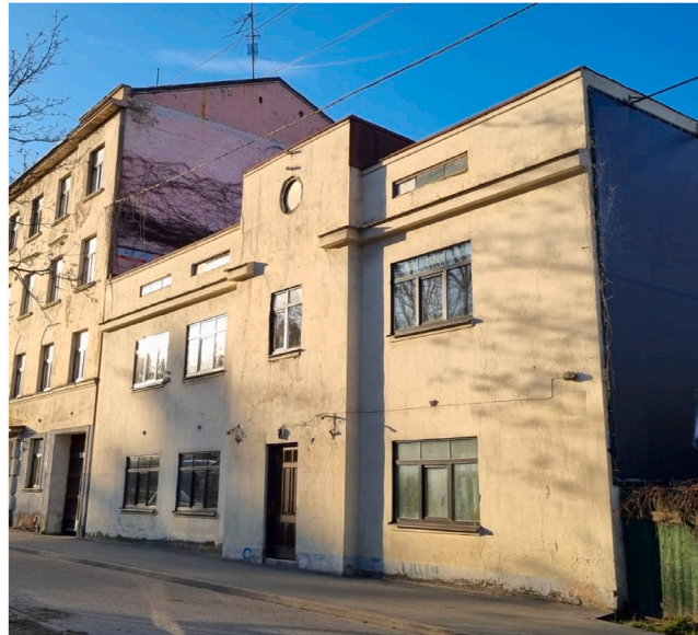
Fig. 1. A wooden multi-story building insulated from inside with hemp blocks.
