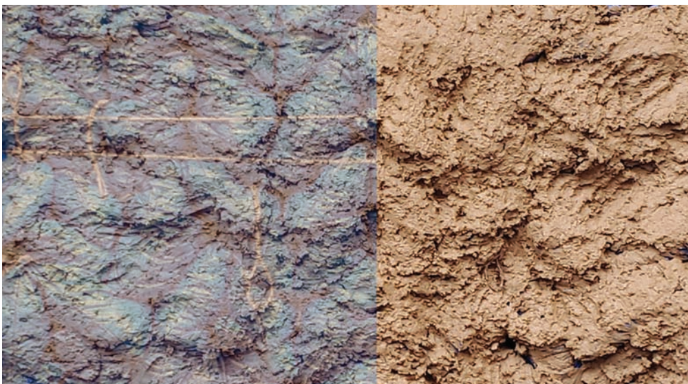
◁ Figure 11. The alternate earthbag geometries in the Bi-cinch wall resulted in a bumpy textured earth surface when rendered with clay plaster.
