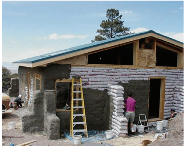
△ Figure 2. Applying plaster to an earthbag home. (Credit: Kelly Hart.)
