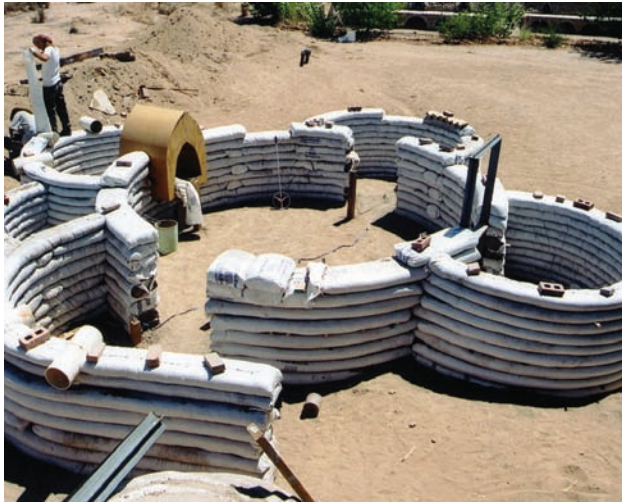
△ Figure 1. Construction of the Eco-Dome. (Credit: CalEarth Institute.)
