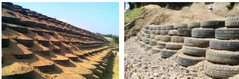
Fig. 16. Representative images of retaining walls reinforced with ELTs (reprinted from Ref. [146]).
