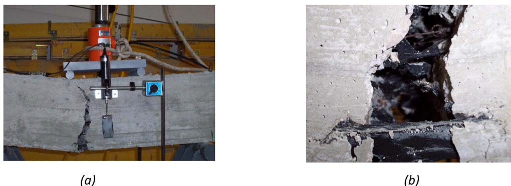
Fig. 4. (a) Rubberized concrete beam after the cracking and (b) particular of the cracked section of the beam (reprinted from Ref. [37]).
