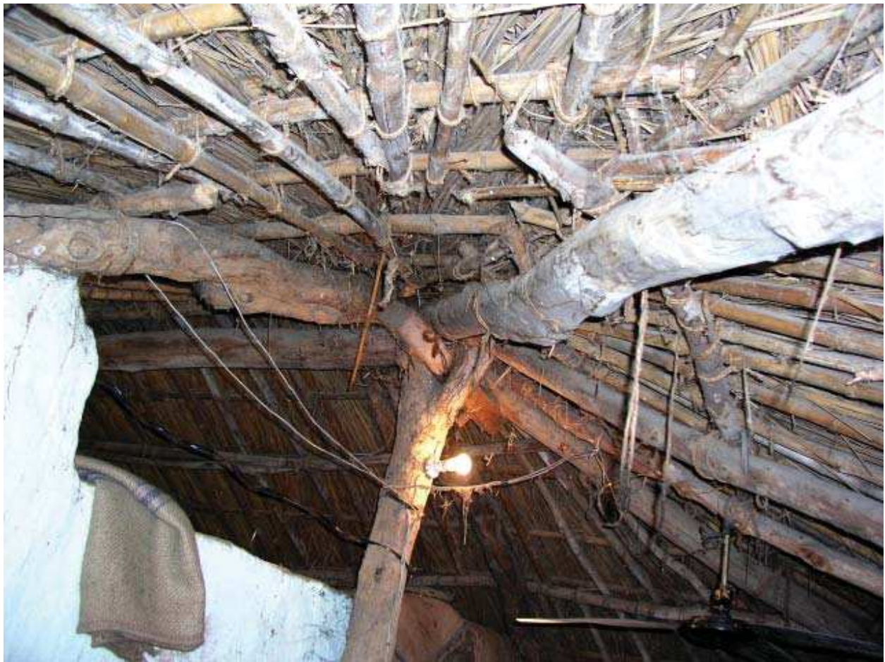
Figure 8. An inside view of a thatched roof. © OC Handa.
